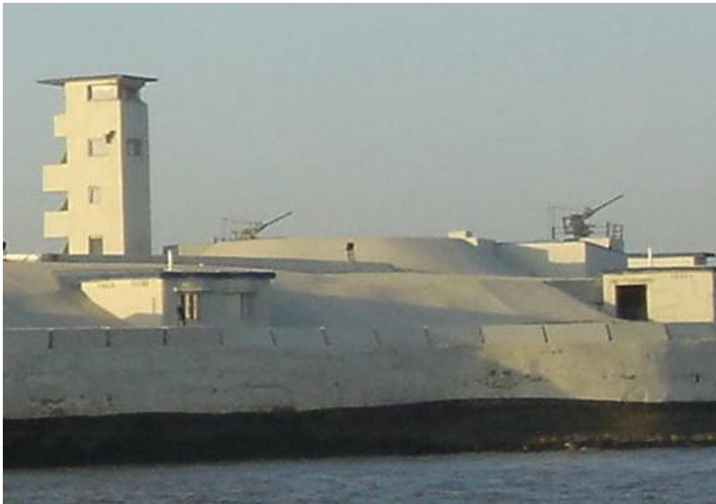
Open L-60 turrets at Middle Ground Coastal Battery. They are dually useful for coastal and anti-aircraft defence. (via Panaramio.com )
